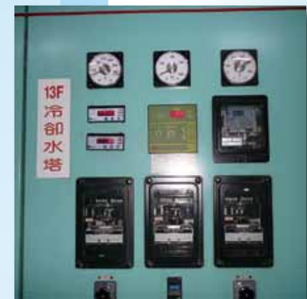
數位水質監控藥劑添加系統 Digitalization of Water Quality Control and Chemical Administration System
